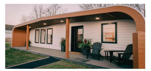
Exhibit 4: A 600-square-foot prototype of the first 3D printed bio house
